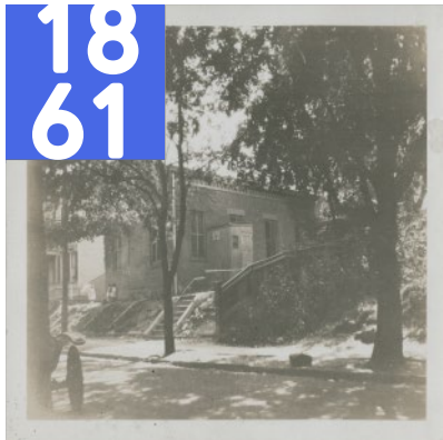
NEW SCHOOLHOUSE CONSTRUCTED (IMAGE: 2; SOURCES: 5, 6)
